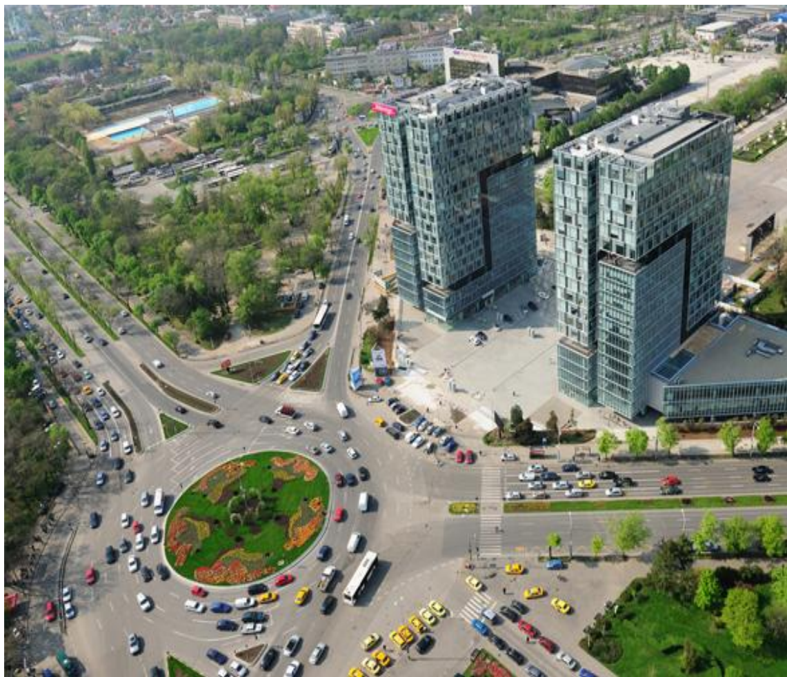
City Gate Towers, Bucharest
