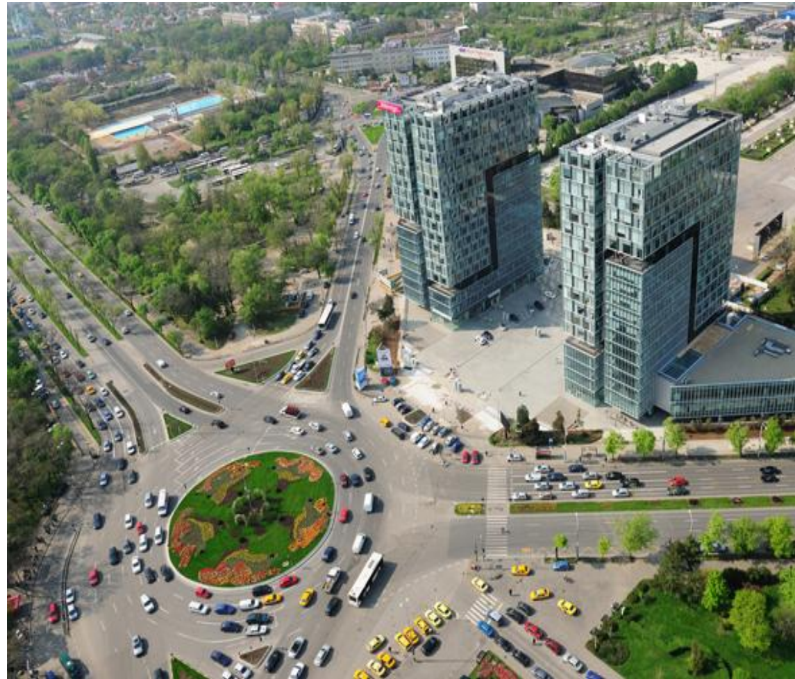
City Gate Towers, Bucharest
